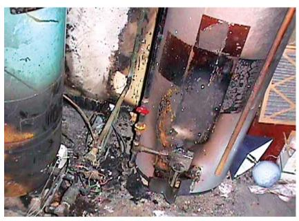
An exploded water heater as a result of improper installation. The Energy Commission provides guidelines for proper and safe water heater installation to prevent accidents like these.
